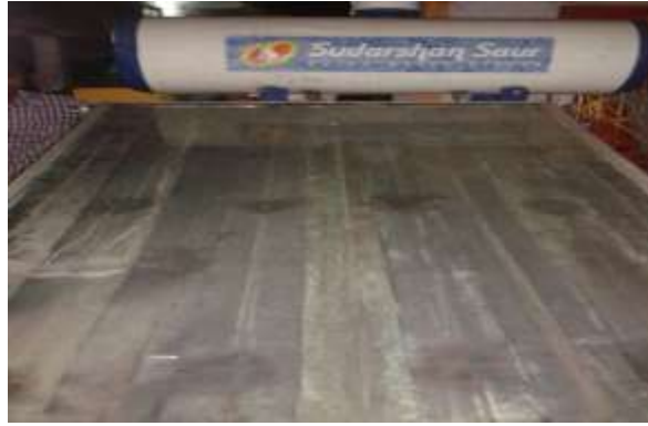
Fig.2.1 Solar Flat Plate collector water Heater with straight riser tube
